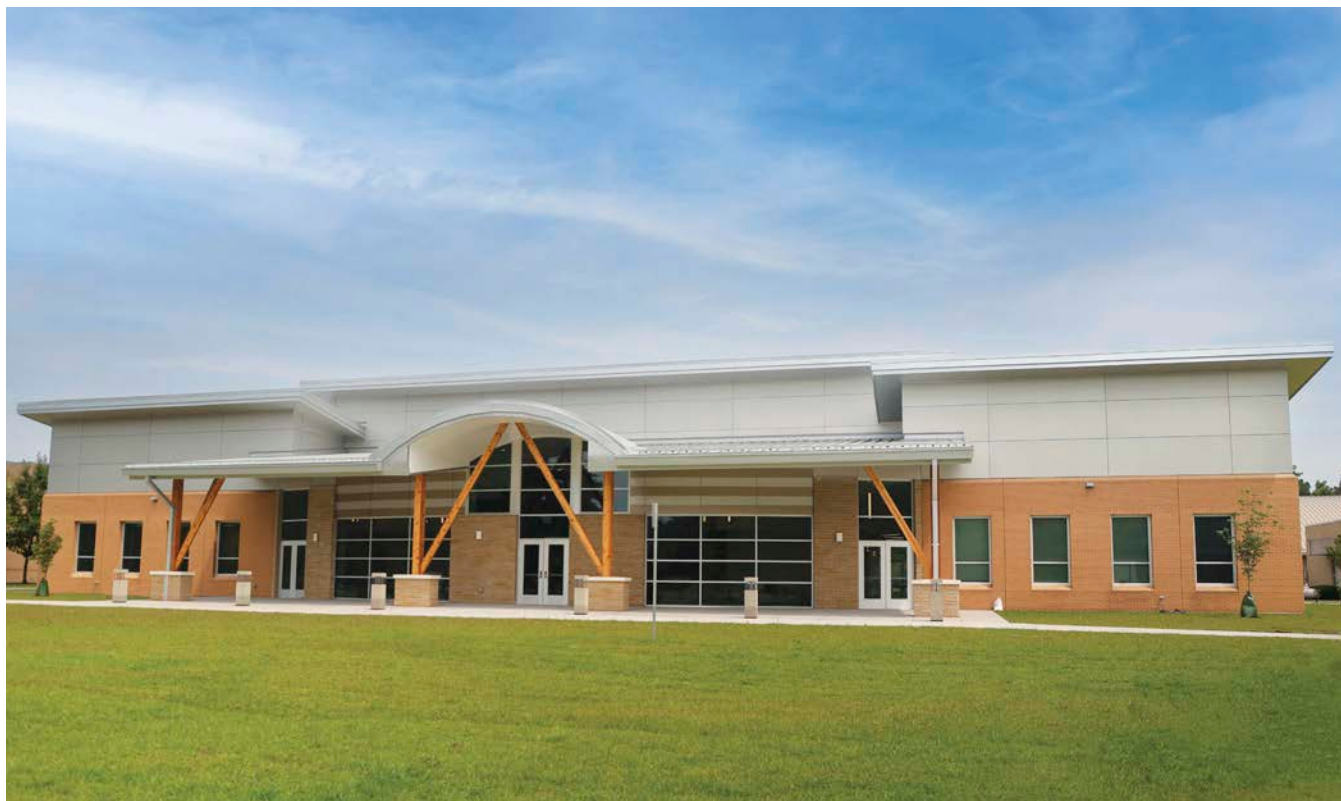
The College's new Corporate Training Center will serve as a community hub for professional development.
